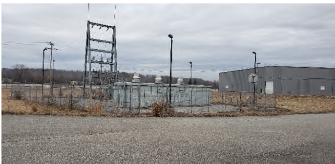
3.) Looking north, remaining transformer station and warehouse
