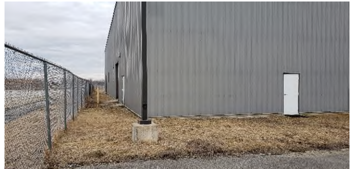
4.) Looking northeast, remaining warehouse
