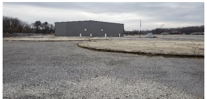
5.) Looking southwest, other remaining warehouse and former tank pads
