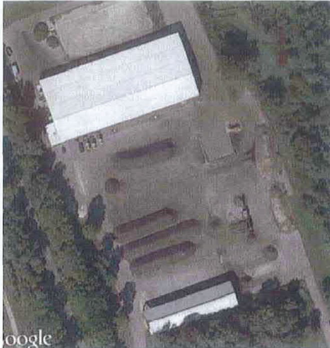
Outdoor windrow type Curing piles adjacent to enclosed Compost Facility (left). Typical Trommel Screen operation (below)
