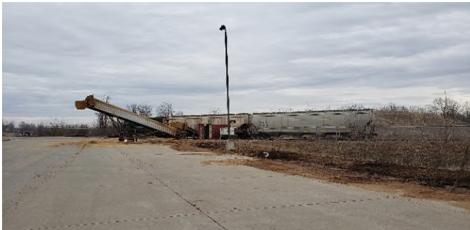
8.) Looking northeast, grain processing equipment
