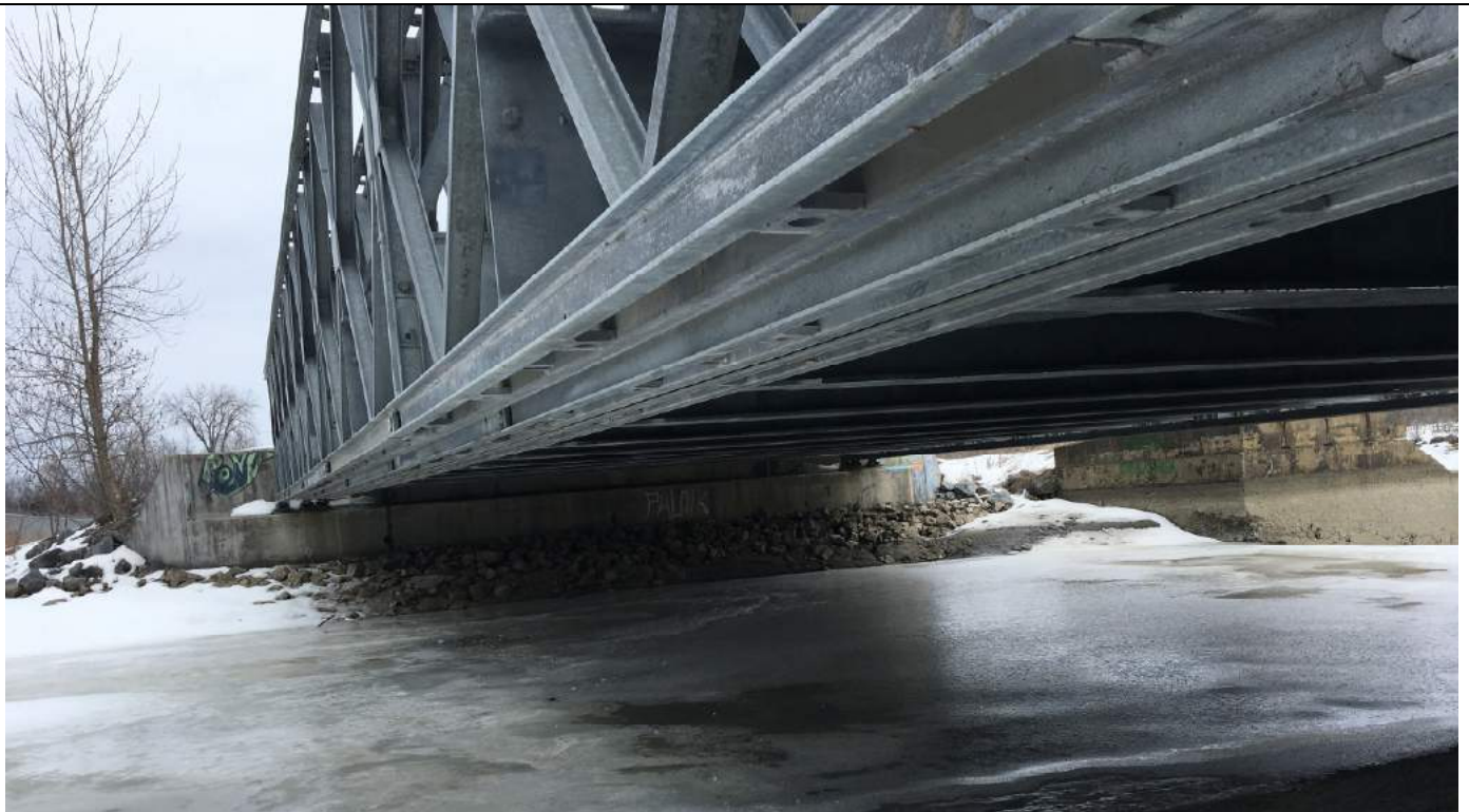
Photo 4 – North Abutment, looking north from south end underside of bridge
