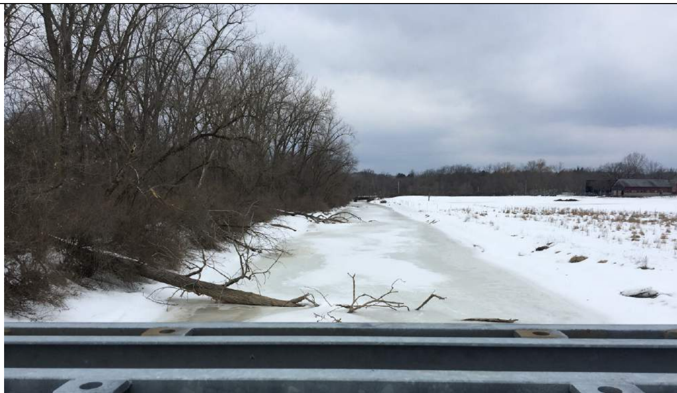
Photo 6 – Feeder Canal, looking west from bridge
