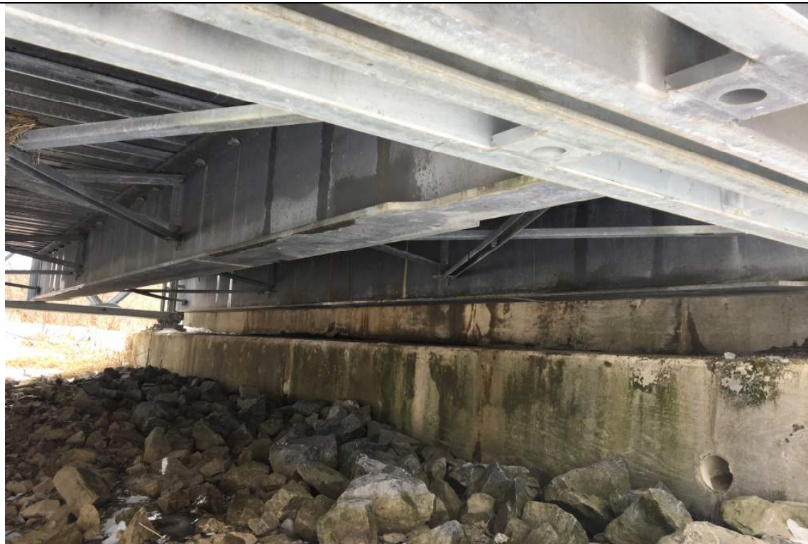
Photo 5 – South Abutment, looking south from underside of bridge
