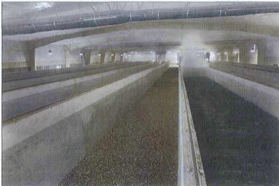
Agitator working in bay next to empty bay
