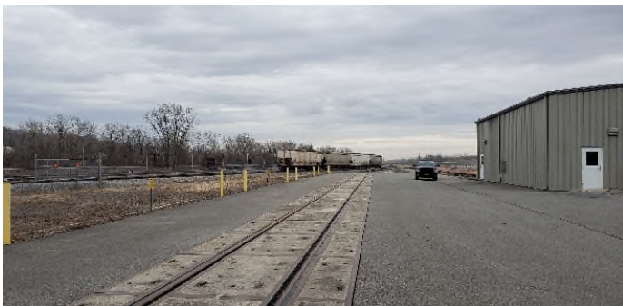
2.) Looking northeast, rail lines
