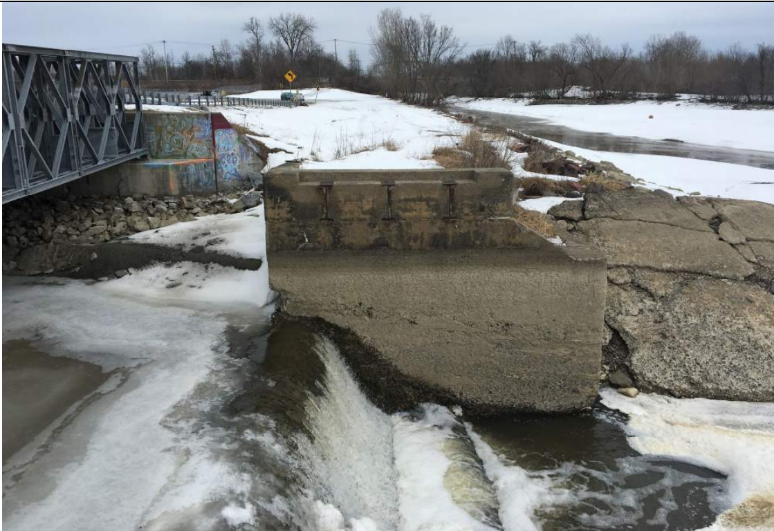
Photo 8 – Canal Spillway/Dam structure downstream of bridge, looking north
