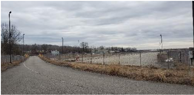
1.) Looking north- northeast, rail line and former dewatering areas
