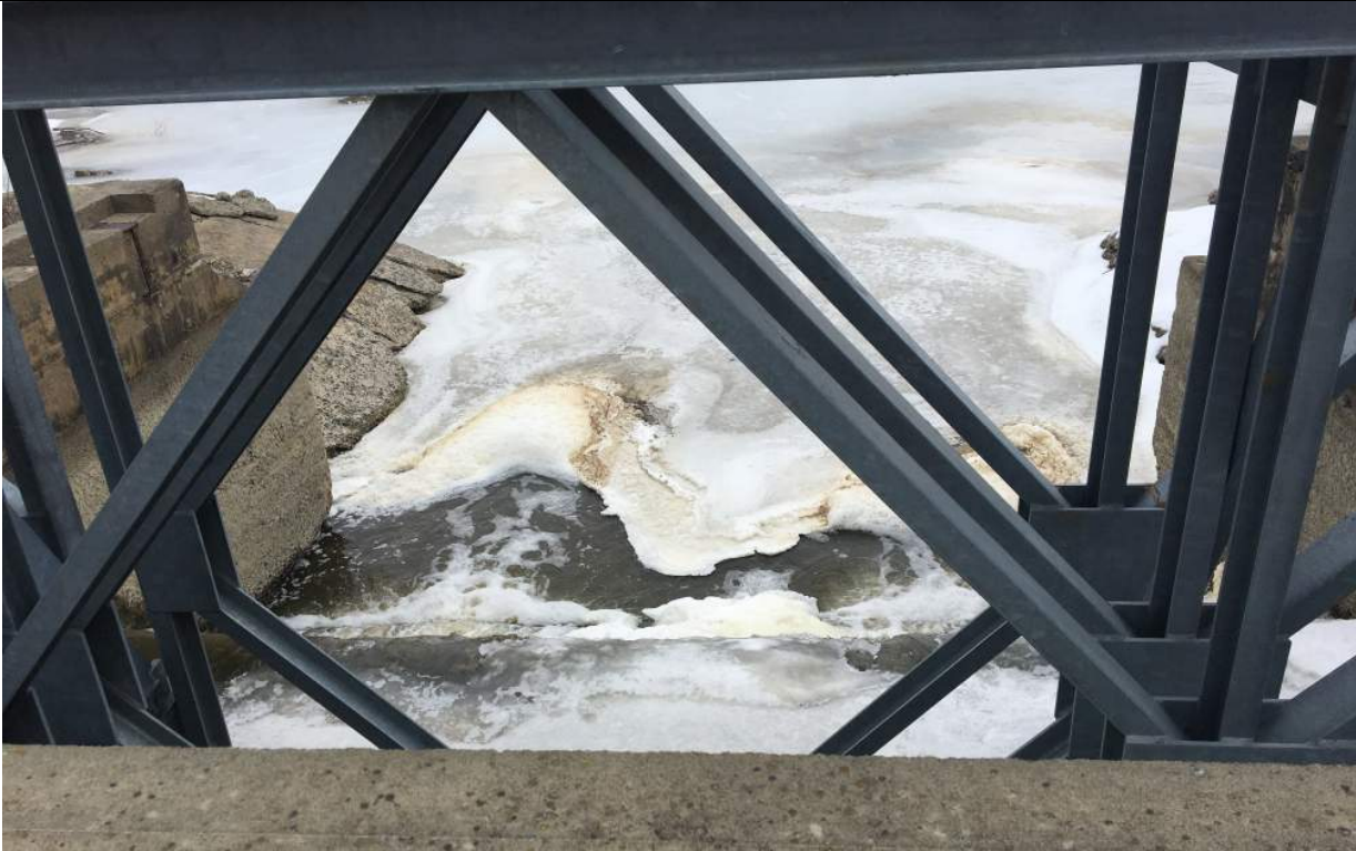
Photo 7 – Feeder Canal downstream from bridge, looking east
